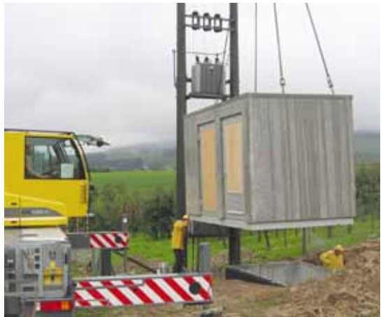
Montage Transformatorenstation Stiigere, Freienwil
